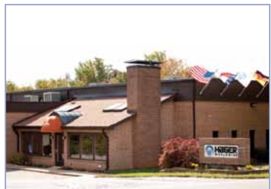
Hager Worldwide Corporate Office Hickory, North Carolina
